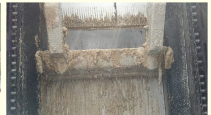
LIFT STATION WELL WITH FLOATING GREASE
