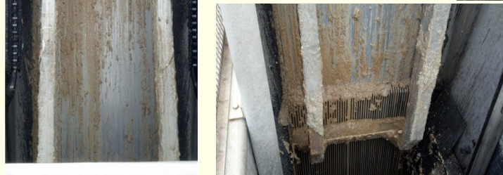
SEWAGE SCREEN AND FILTER'S INSIDE OF THE PLANT ARE COVERED IN GREASE & OIL
