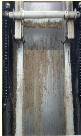
SEWAGE SCREEN AND FILTER'S INSIDE OF THE PLANT ARE COVERED IN GREASE & OIL
