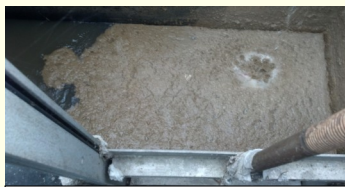
LIFT STATION WELL WITH FLOATING GREASE
